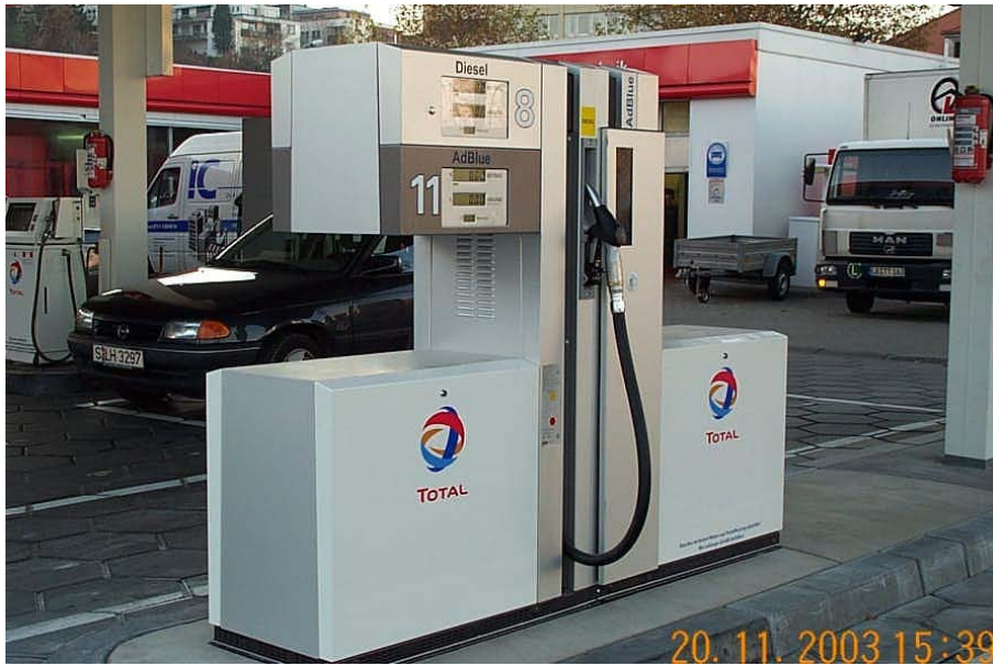
Figure 4: Service Station TOTAL, Stuttgart Ulmenstraße
